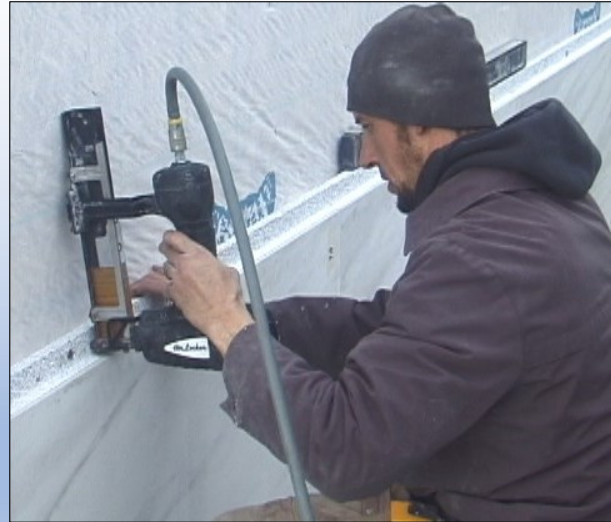
Screw/washer or Wide Crown Staples through the foam attachment
